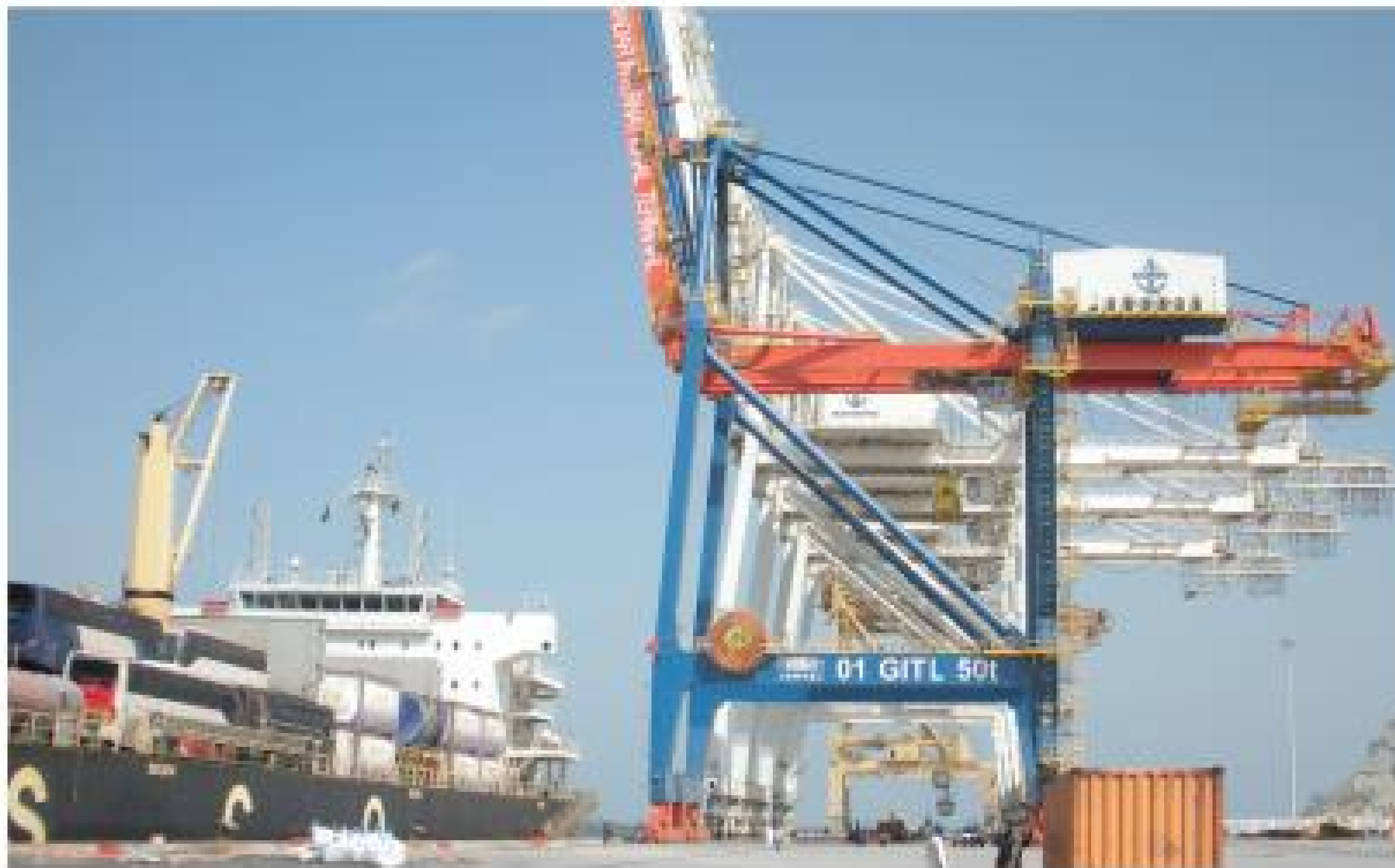
Gwadar Port, which is the apex of the CPEC project, is strategically located in the Arabian Sea. Photo/Supplied
