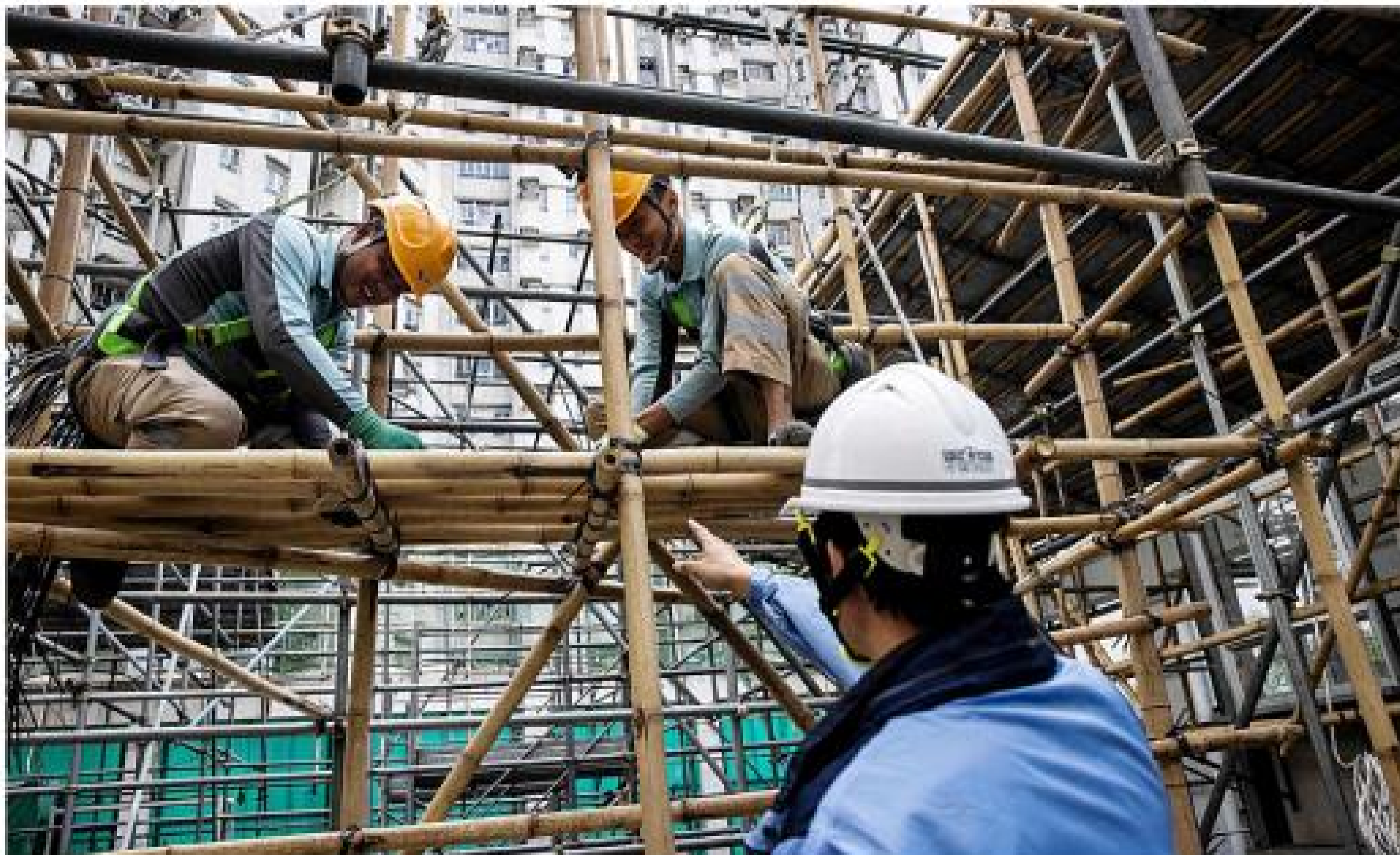
Structure Students at the Hong Kong Institute of Construction receive instructions from their instructor during a bamboo scaffolding class. The world's most skyscraper-laden metropolis is also one of the last remaining major cities to use bamboo scaffolding for modern construction and building repair.
