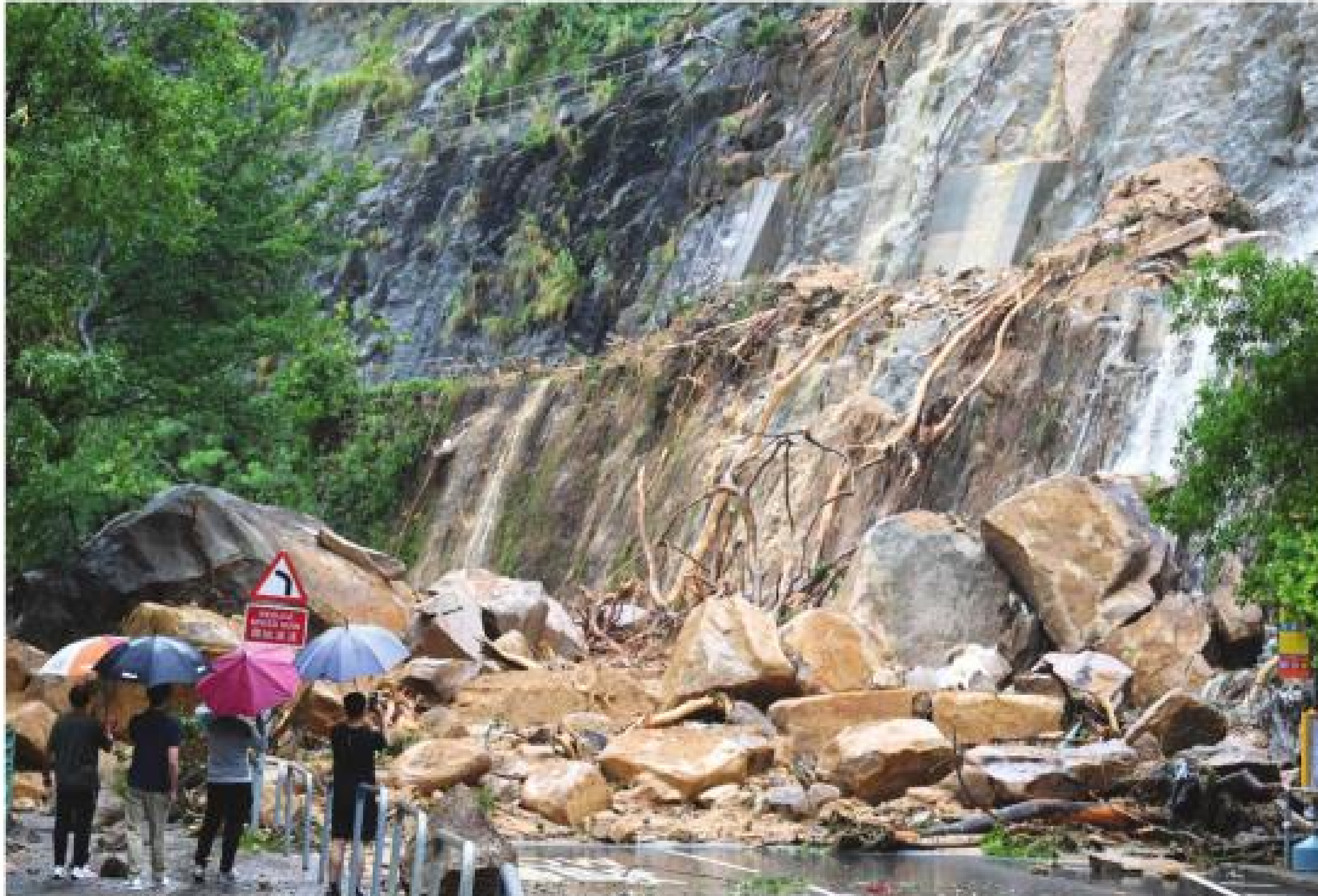
Plainclothes officials and police look at a landslide covering a road at Yiu Tung Estate in Shau Kei Wan in Hong Kong on Friday following heavy rains. AFP
